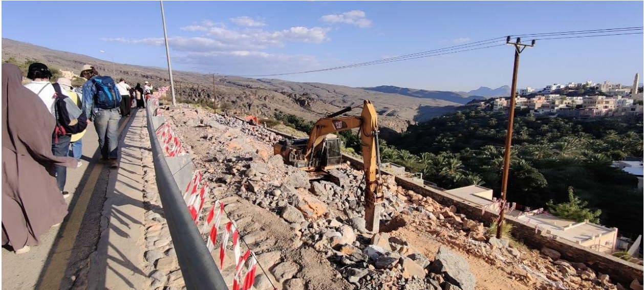
Image 5: Construction of new parking lots, Misfat Al Abriyyin. Credits: Leon Wiesemann.
